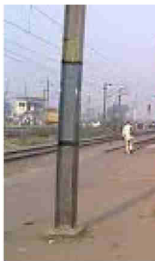
Noida: The Greater Noida (GreNo) Authority has undertaken the task of restoring the Dadri railway road. It will soon issue the tender process. Work is likely to begin next month.
